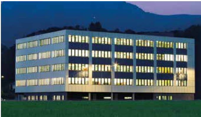
Leister Technologies AG, factory, Samen, Switzerland
