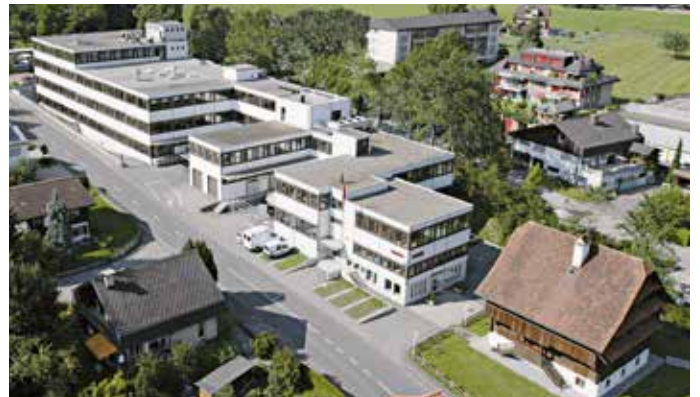
Leister Technologies AG, factory, Kaegiswil, Switzerland
