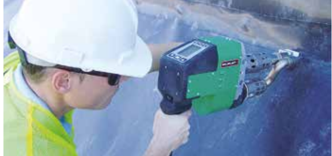
The powerful WELDPLAST S4 at work.
