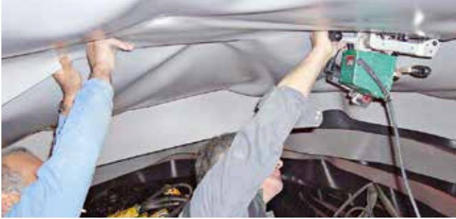
Comet operating in the tunnel ...
